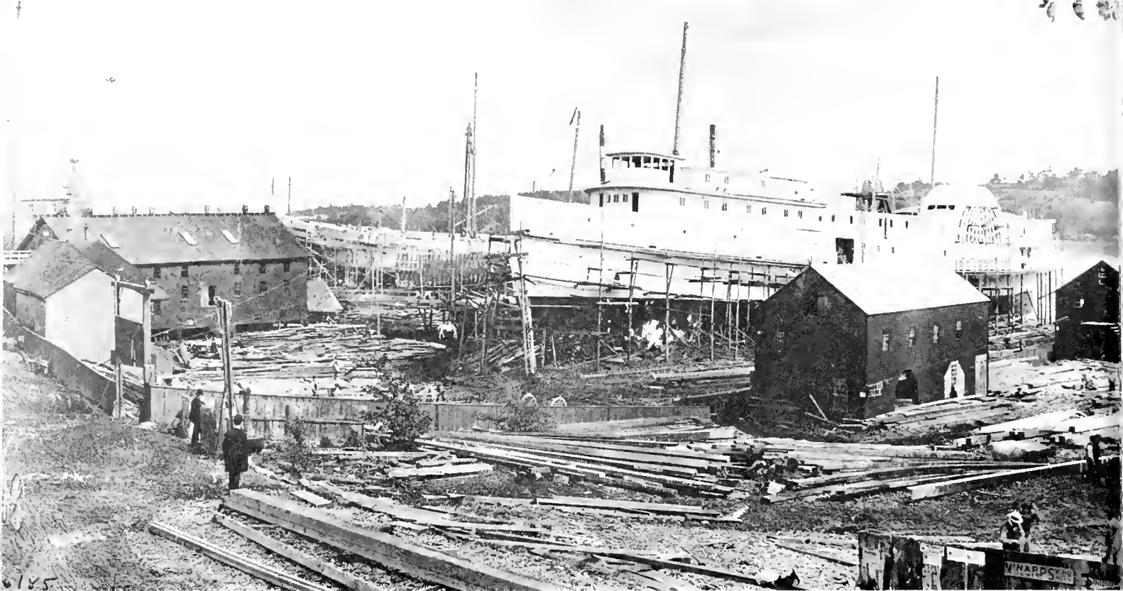
SHIPYARD OF THE NEW ENGLAND SHIPBUILDING COMPANY, Bath, Maine, in 1860. Under construction is the steamer Portland , lost with all hands November 26-27, 1863 in a storm that became known as the "Portland Gale." A 3-masted coaster is building in background. (Smithsonian photo 44792-c.)
